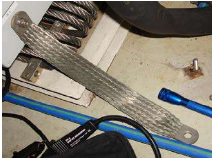
Earthing check R < 2.5 \text{ m}\Omega or 10 \text{ m}\Omega
